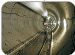
Dewatering of Basement Water
